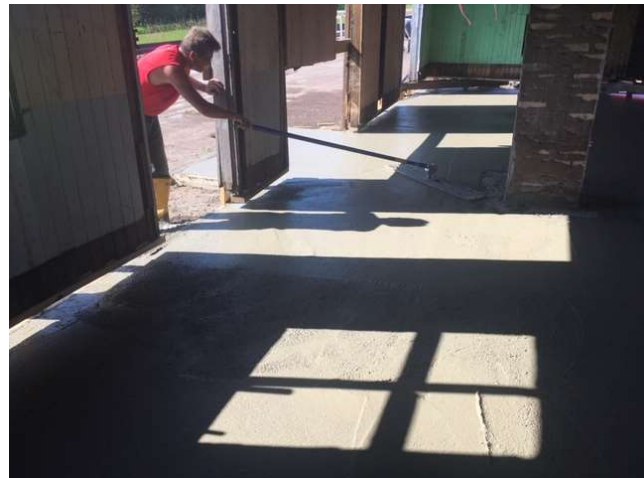
Brad Reitan finishes the depot slab
