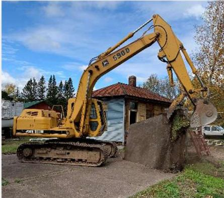
The skilled backhoe operators from Ostman Trucking & Excavating made quick work of carefully removing old depot apron. The space left was filled with Class 5. Photo: Paul von Goertz
