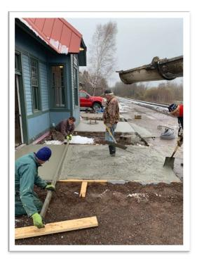
*Photo on left*, Mike Ostman Trucking and Excavating did a very professional job removing the cracked and heaved original concrete apron, without damaging existing usable sections along the railroad right-of-way. *Photo on right*, volunteers screed freshly-poured concrete.
