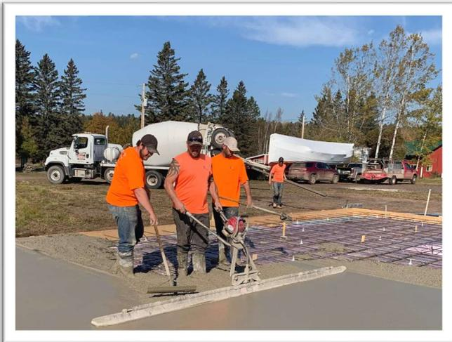
The mood was almost festive for the sidewalk superintendents who were present on October 21 to see 32 cubic yards of concrete poured to form the 23' x 46' commercial fishing exhibit slab. The concrete workers (photo left) from Primetime Concrete on Old North Shore Drive smoothed freshly poured concrete. Three truck loads were required. Primetime was good to work with, met our timelines, did the
